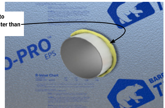
Step 2: Apply spray foam to fill gaps.
