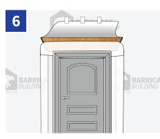
Install and shim door into rough opening per manufacturer's instructions. When using sealants or primers, be sure Barricade branded (or compatible) sealant is used.
