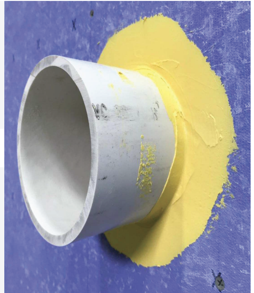
Apply additional Barricade Liquid Flashing
